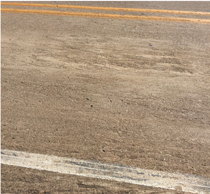
PHOTO 1 Description Typ. Cracking in Deck.
