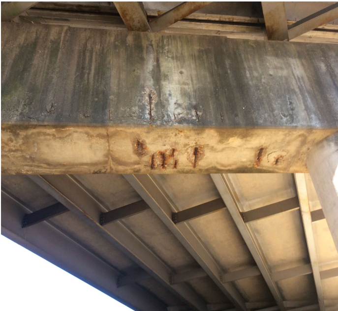
PHOTO 1 Description Delam, Cracking & Spalling W / Rebar Exposed in Bk. & Bt. Faces of Cap 4. Spalling due to Rebar too close to Surface.
