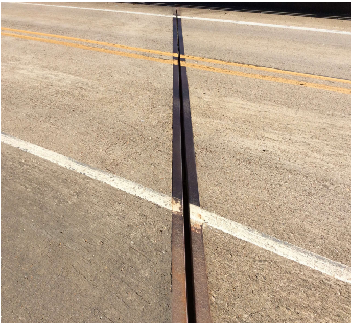
PHOTO 1 Description Seal Failed at Joints.
